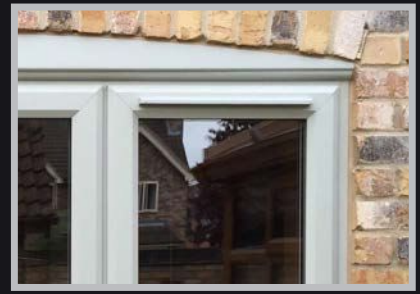
Trickle vent through a Rebated Sash
