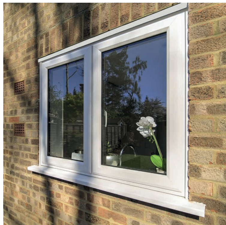
Concealed Ventilation installed through the outer frame
