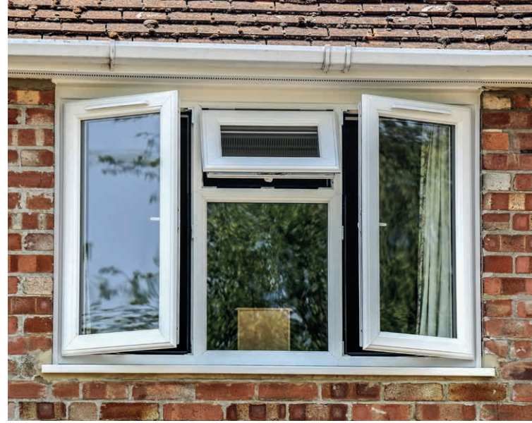
Trickle Vents installed through the window sashes
